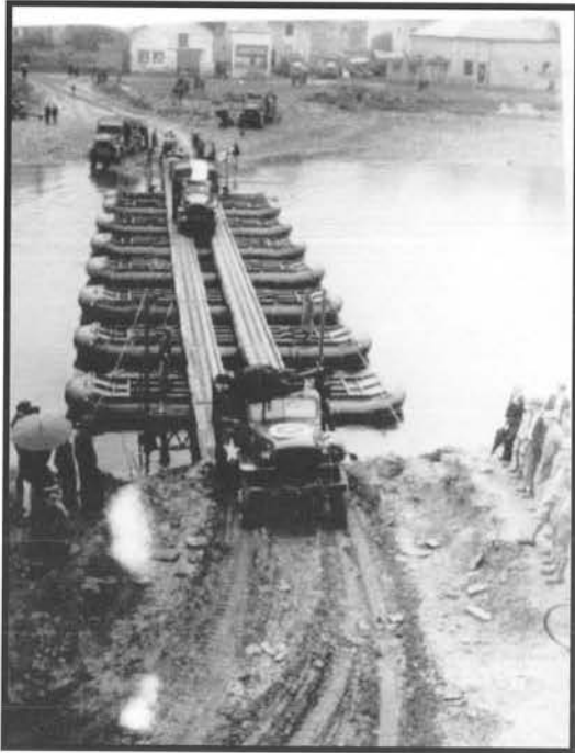
Yank trucks of the 4th Infantry Division Engineers cross the Muse River at Montharme France by this Engineer Pontoon Bridge, 8 Sep 1944, France.
