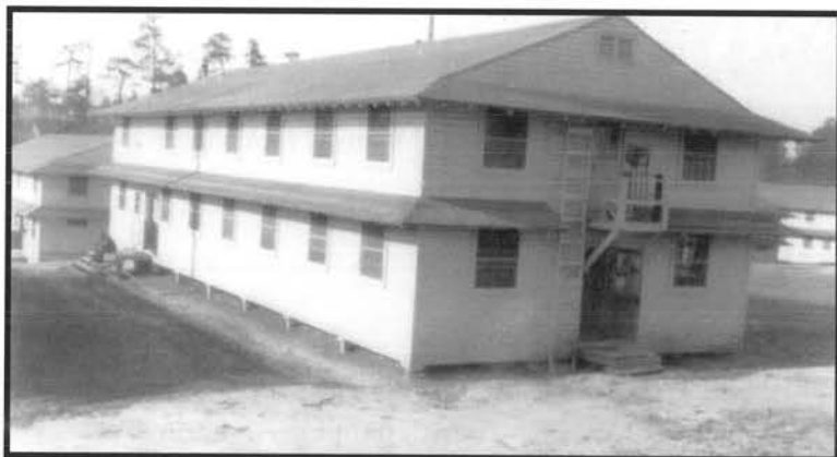
Number 4 barracks, Fort Benning, Georgia, 1941
