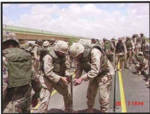
Engineers construct a floating bridge across the Tigris River at Tikrit until the partially destroyed permanent bridge (background) can be repaired. 28 April 2003
